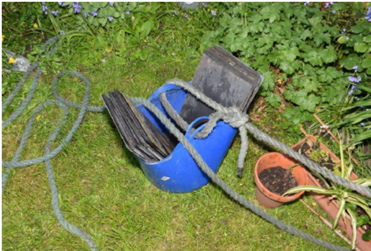
Image of unsuitable and untested lifting accessory
