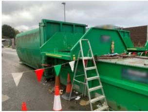
A HSE inspector identified unrestricted access to the controls and to dangerous parts of the machines
