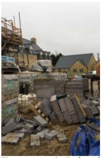
The company had also failed to ensure that wooden pallets in a suitable condition were used for the storage of construction materials
