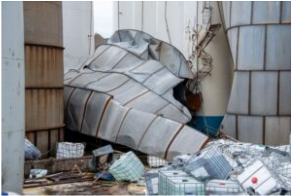
The 700-tonne tank was more than 30 years old
