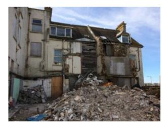
During a proactive inspection, the Health and Safety Executive (HSE) identified that the former hotel was being refurbished and partially demolished whilst ACMs remained in-situ. Some of these ACMs were licensable products (e.g. asbestos insulating board which contains amosite). Due to the extent of the spread of asbestos dust and debris throughout the building and the lack of adequate control measures, workers and visitors to the properties were at risk of exposure to asbestos fibres.
