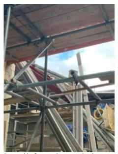
Remedial work was being carried when a steel beam and a block of the first floor collapsed
