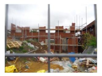
There were also reports that bricks had fallen from the scaffold, and the building's gable end wall apex section had at one point collapsed onto the neighbouring property. Despite HSE serving a number of enforcement notices and notification of contravention letters, serious breaches of health and safety law continued and there was a failure to comply with the enforcement notices.
