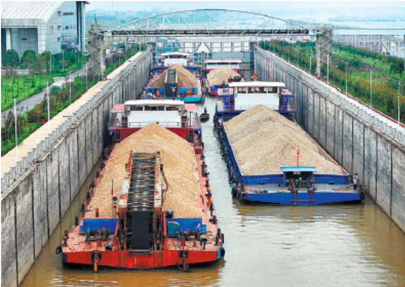
A navigation lock in operation in Xiangjiang River in Changsha, Hunan province. [Photo/Xinhua]
