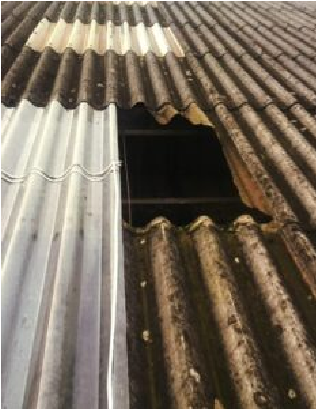
The roof Billy had been working on
