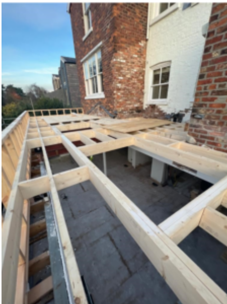
Work area where the incident occurred
