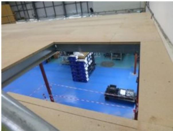
An investigation by the Health and Safety Executive (HSE) revealed that the contractor failed to adequately plan, manage and monitor the construction work, so as to ensure that appropriate methods to prevent or mitigate a fall during the construction work, were in use.
