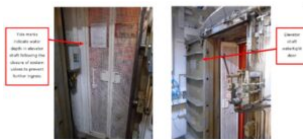
Figure 11 – Lift Entrance and Water-tight Door in P-M-12
