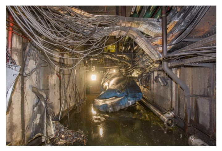
A HSE investigation found that a flammable atmosphere developed within the accumulator as hydraulic lubrication oil was being drained from it. The flammable atmosphere was ignited by an electric heater within the accumulator.
