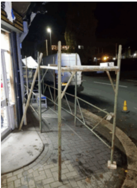
The scaffolding tower without edge protection
