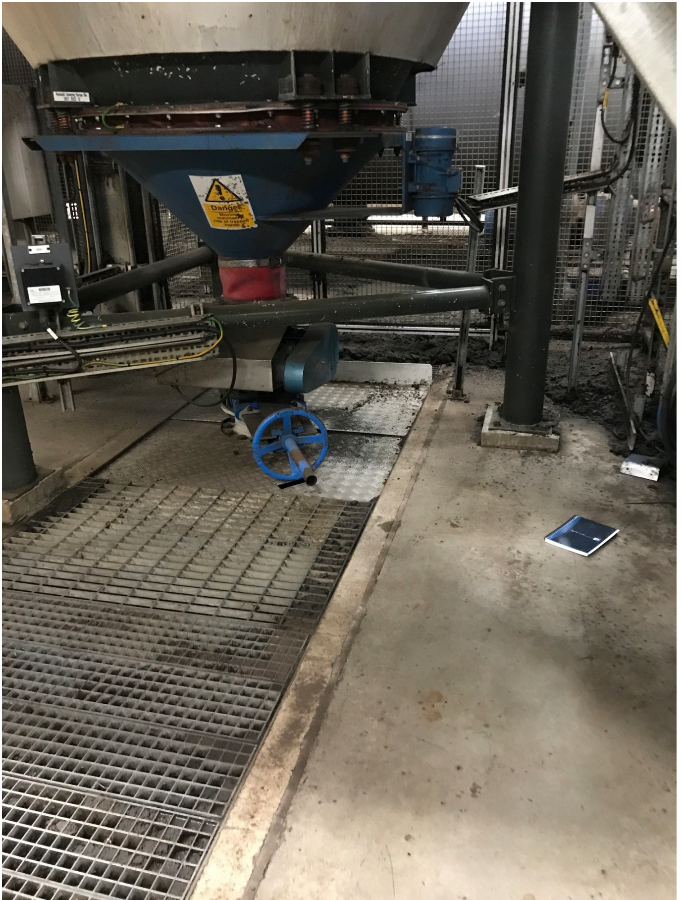
The surge hopper onsite
