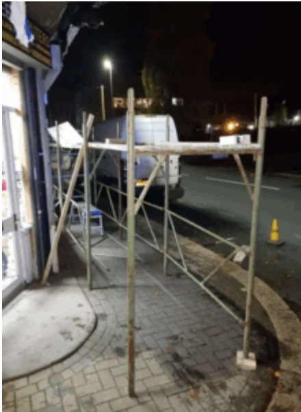
The scaffolding tower without edge protection
