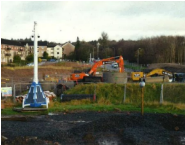
The construction site adjacent to Glenkirk Drive
