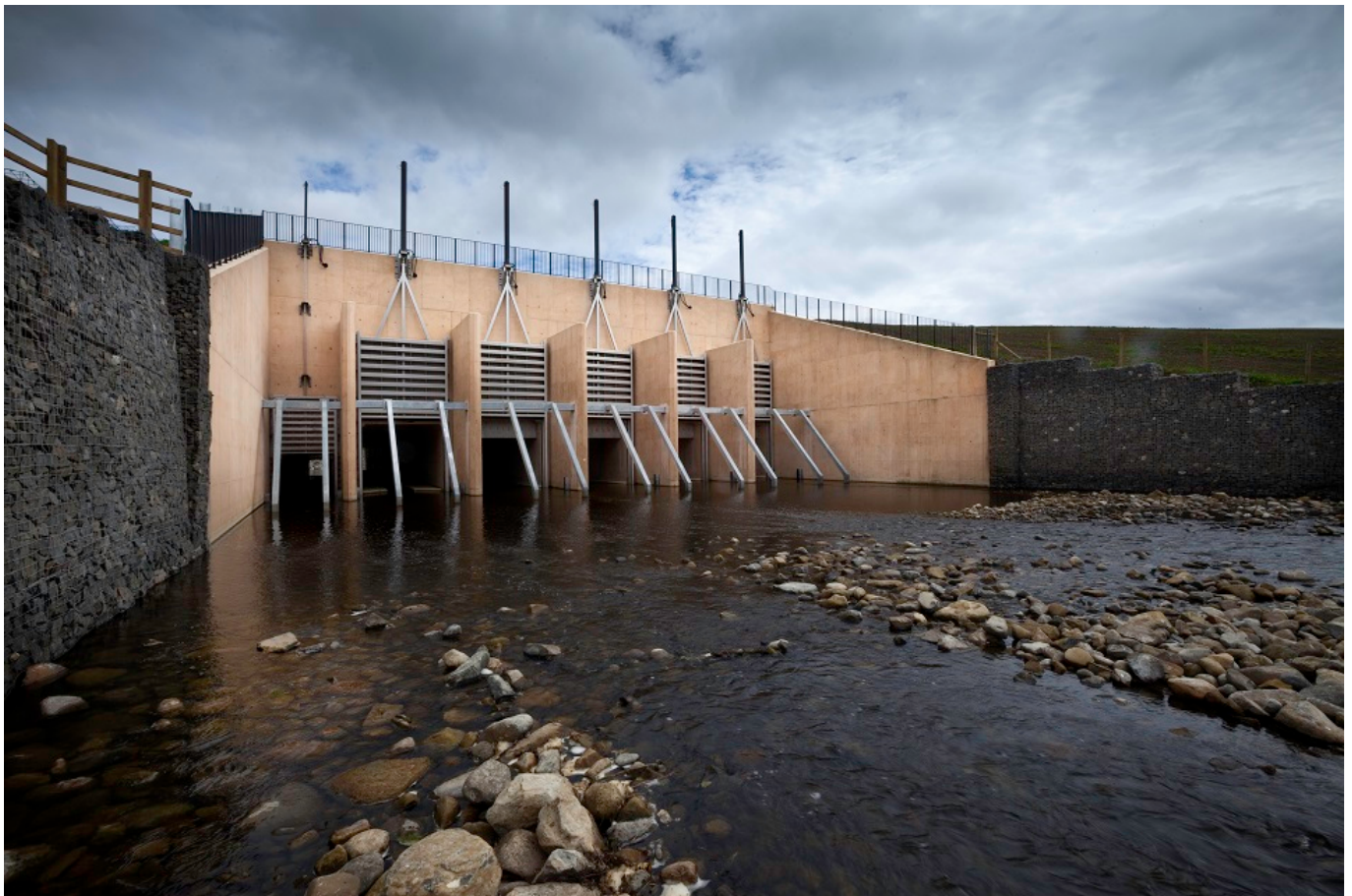
The large dam at Mitford
