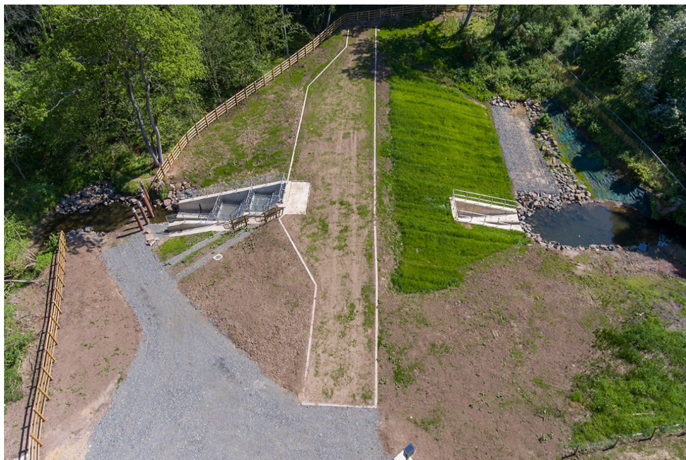
Cotting Burn dam aerial image
