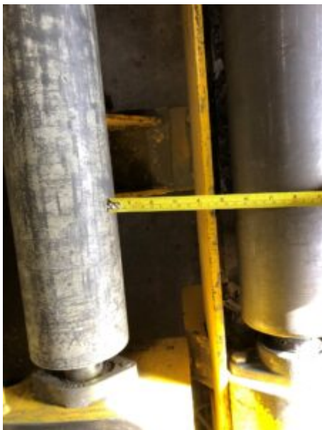
Photo of gap in roller deck pre-accident
