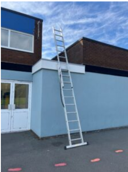
Ladders leading to roof
