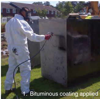
1. Bituminous coating applied
