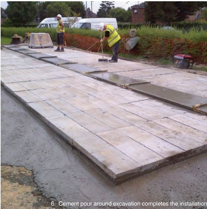
6. Cement pour around excavation completes the installation
