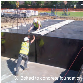
3. Bolted to concrete foundation
