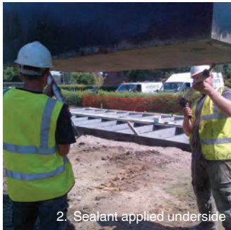
2. Sealant applied underside
