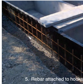
5. Rebar attached to hooks
