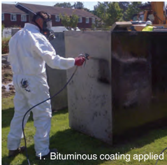
1. Bituminous coating applied
