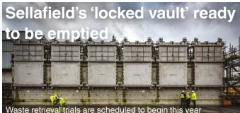
Engineering teams have installed equipment to scoop up and remove material from Sellafield's Pile Fuel Cladding Silo.
